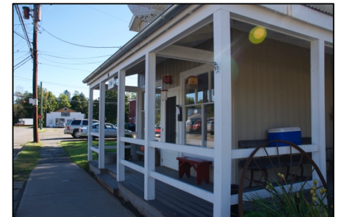
Above (top to bottom): Butterfields Cafe on Division Street in Deposit, NY and view of front porch and outdoor seating for the café. While this café is not situated within the Downtown business district, it is located on an important gateway to Downtown. The signs, large windows and nice presentation of the exterior and interior of this restaurant, coupled with its menu, make for an inviting culinary destination that has broad appeal.
