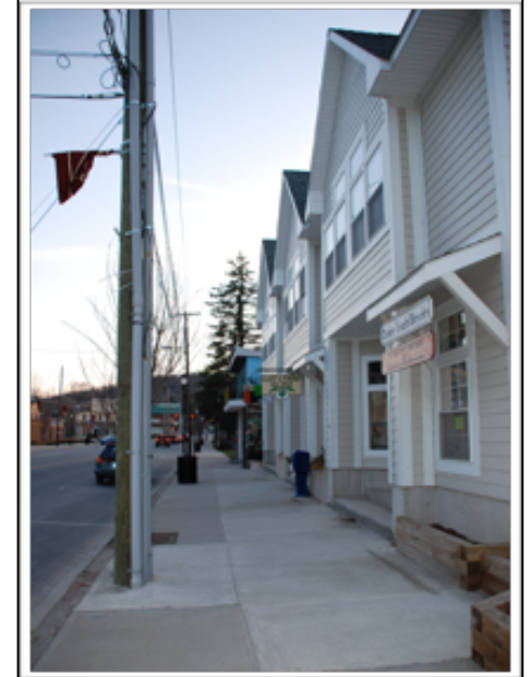
Above: This infill building was constructed on Main Street in Livingston Manor, NY, which is an area that is very prone to periodic flooding. It was constructed so that the bottom of the lowest horizontal structural member of the lowest floor (excluding the pilings or columns) is elevated to or above the base flood level and the foundation and structure attached thereto is anchored to resist floatation, collapse and lateral movement because of wind and water loads acting simultaneously on all building components.
