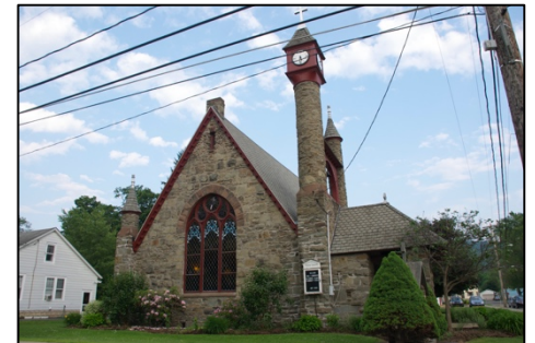
Above (top to bottom): Painted Lady (i.e., three or more colors that embellish the architectural details) Victorian home that is well preserved; eclectic home on Second Street with a variety of architectural influences that is showing signs of needed repairs and Christ Episcopal Church on Second Street, which is adjacent to Monument Square. The structures above are architecturally significant and eligible for listing on the National Register of Historic Places.
