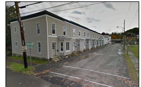
Above (top to bottom): View of well-maintained sidewalk segment in front of the State Theatre in the heart of the Downtown business district along Front Street; view of well-maintained ADA compliant sidewalks along both sides Court Street [between Front Street and Second Street] and view of poorly maintained sidewalks and drains along Church Street [between Front Street and Second Street] that are a deterrent to pedestrian travel. This Plan support complete street enhancements along this segment of Church Street.
